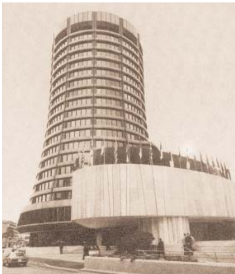
The BIS: Bank for International Settlements in Geneva.
